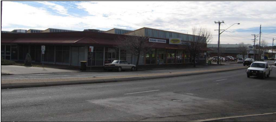
View of subject land from Byng Street looking northeast
